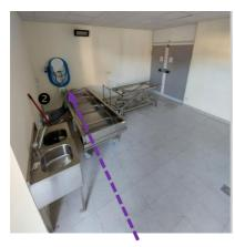
Version with stretcher and central extraction - In this version the air will be captured at the end of the tank ②
